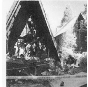
Lake Arrowhead, California Fire Destroys A-Frame Home
